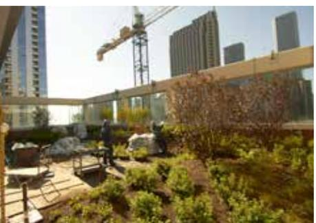
To complete the greenroof design, a walkway and hardscape area, constructed of pre-cast concrete pavers, was integrated into the various planted areas. CETCO also provided several vegetated trays and UV resistant, white, reflective PVC membrane for the penthouse portion of the greenroof. As a single source provider of greenroof solutions, CETCO's products are designed to work together, in multiple configurations, to maximize the success of the roof.
