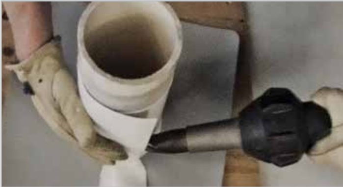
STEP 2. Tack weld PF340 to fit penetration
