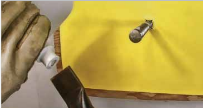
STEP 4A. Heat trimmed PF-150 cut end
