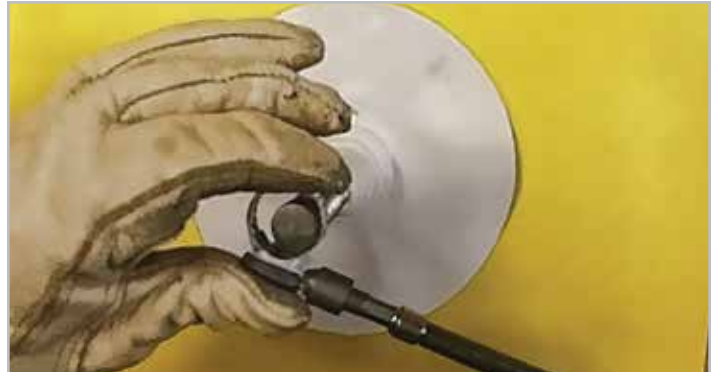
STEP 6. Hose Clamp Loosely Installed
