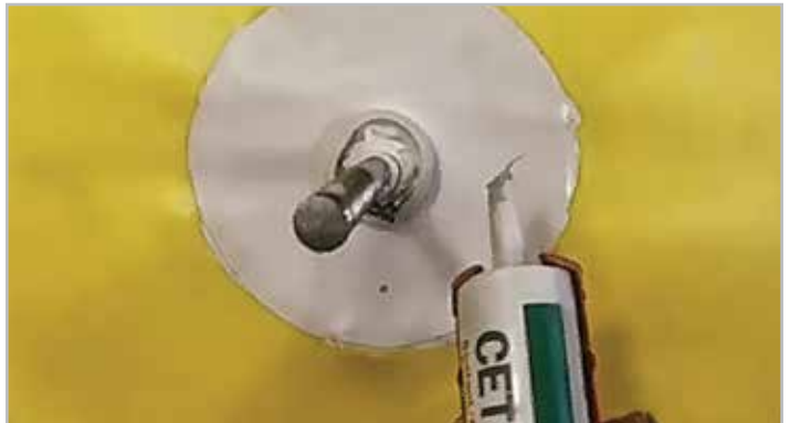
STEP 10. Apply CETSEAL at termination
