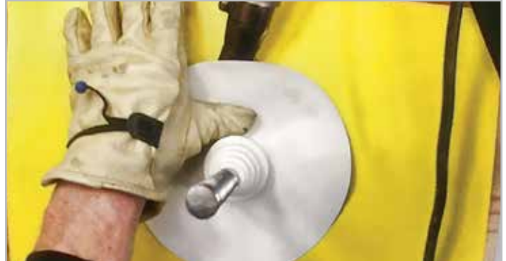
STEP 5. Tack weld PF-150 flange
