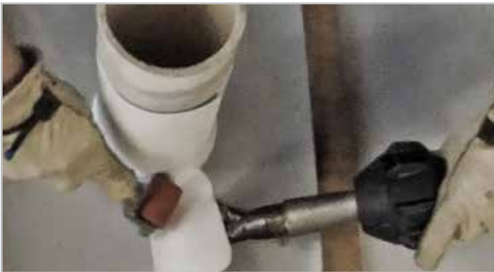
STEP 3. Weld PF340 overlap at base flange
