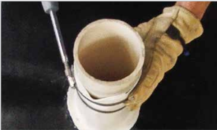
STEP 8. Install second clamp
