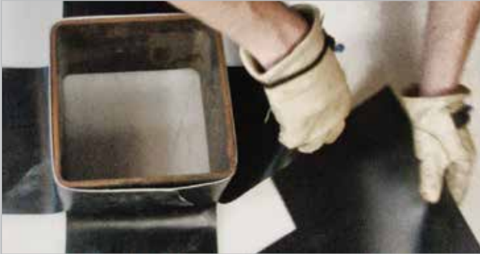
STEP 3. Place corner target patch
