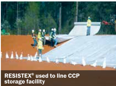
RESISTEX® used in Coal Combustion Landfill Capping, Mallorca, Spain
