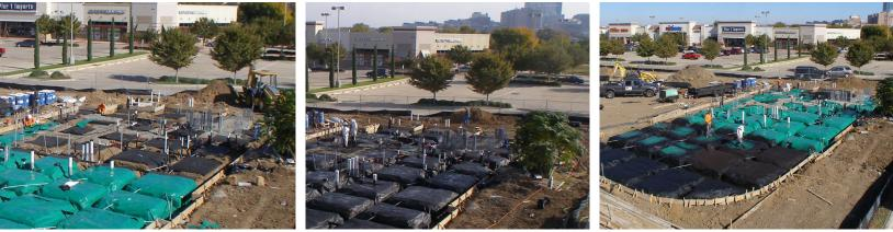
Images (left to right): Installation of the VI-20™ geomembrane with EVOH technology over the low-profile GEOVENT™ gas venting system; fininshed installation of the LIQUID BOOT<sup>®</sup> spray-applied vapor barrier over the VI-20™ geomembrane; in-progress view of the spray-applied barrier being installed over the geomembrane.
