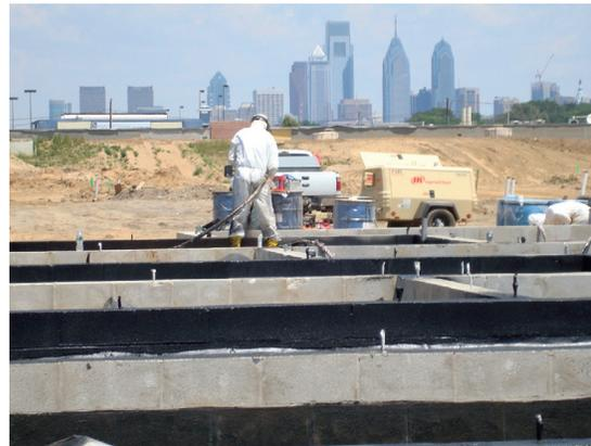
Images left to right: BASEFABRIC™ T-60 provides a uniform substrate to spray the LIQUID BOOT® vapor barrier; the spray-application fully adheres to irregular surfaces, allowing for ease of installation, labor savings, and a gas-tight and seamless barrier; LIQUID BOOT® vapor barrier being installed by a certified applicator on each of the building footprints.
