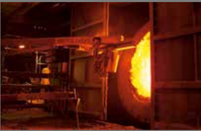
C I – fixed installation For converter
